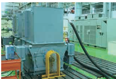
Combined test with inverter drive
