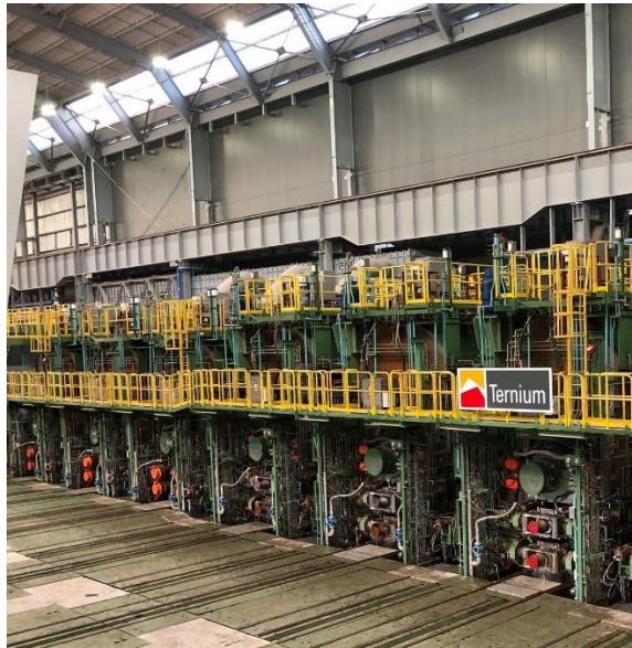
Newly established hot strip mill
